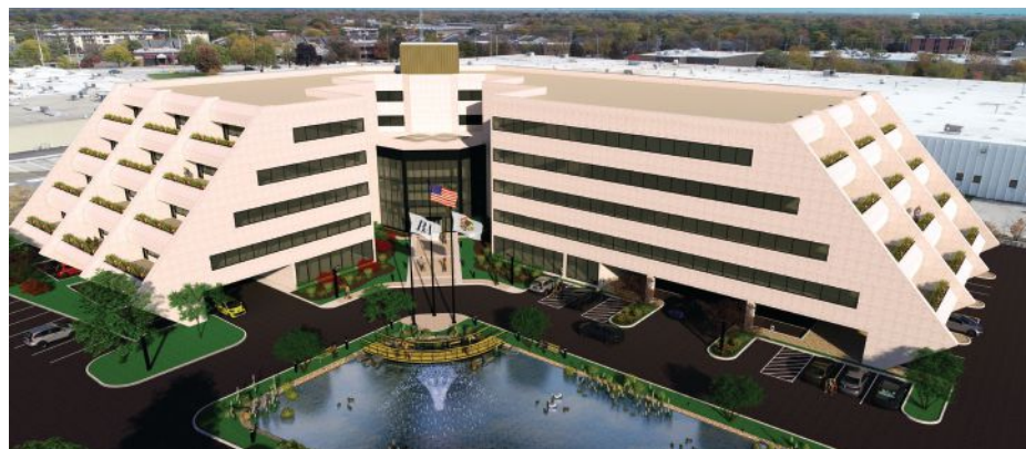
Bradford Allen is transforming the former Daily Herald office building in Arlington Heights, Illinois, into a medical office development named ArlingtonMed.
