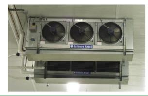
Murphy integrates mechanical systems, building envelope and lighting systems to achieve high returns on beer distributor investments aimed at reducing total energy costs. These ceiling-mounted aircoil evaporators are part of a warehouse cooling system.
